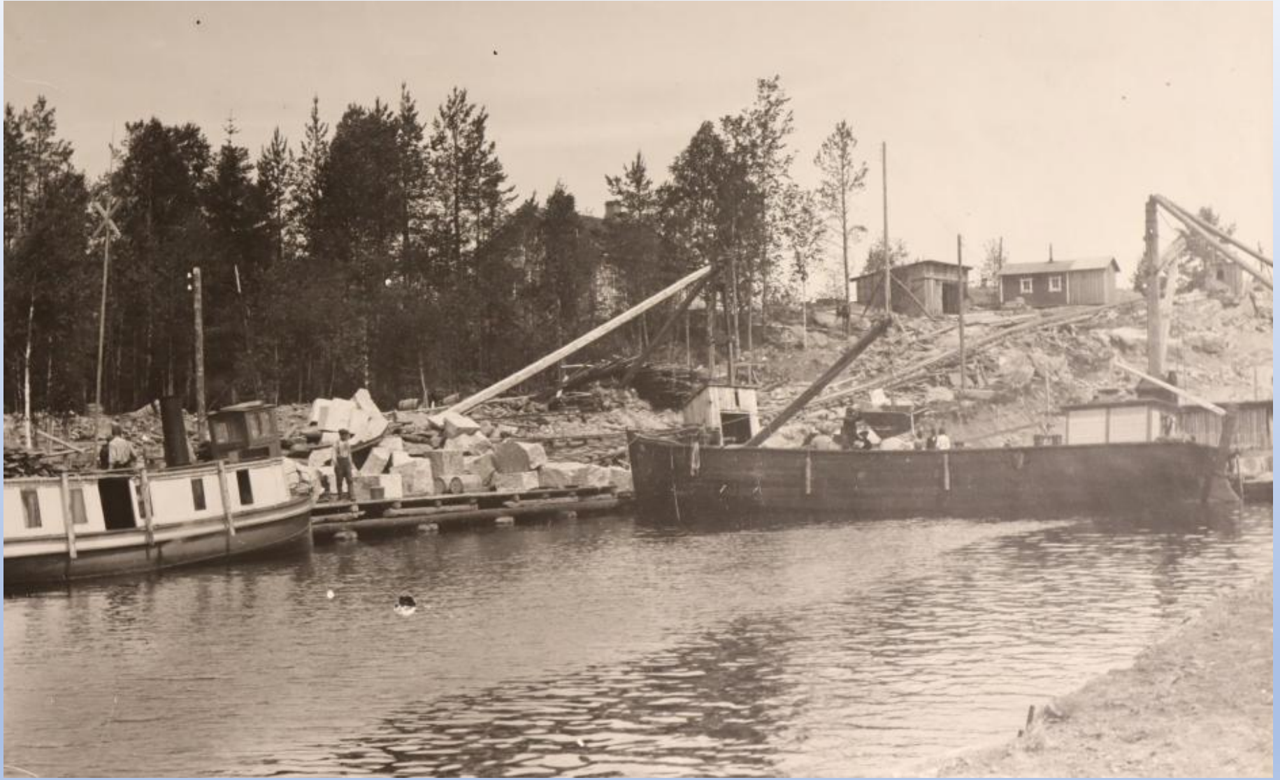
Loading wall- and doorstones from barges to the site
